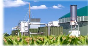
Biomass Power Generation
